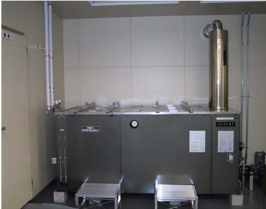
Figure 7. Surface sterilization system using hot water.
