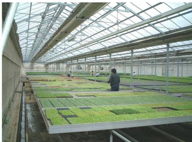
Figure 1. In order to lessen the rapid changes with time in air temperature and relative humidity, a tall greenhouse (6-10 m high) with large air mass is needed for growing short transplants with only about 0.2 m high, which is space inefficient and costly.
